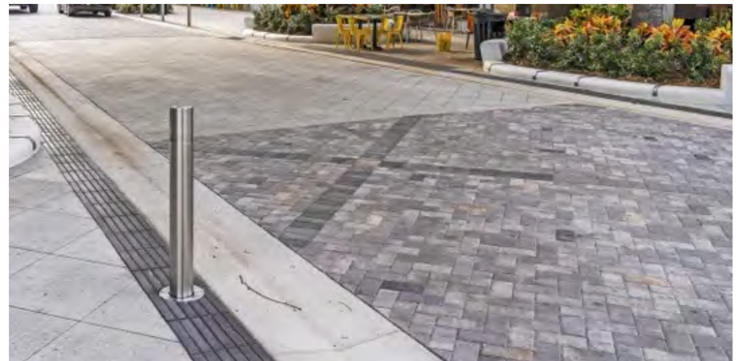
Retractable bollards on Clematis St. - a flexible street in West Palm Beach, FL
