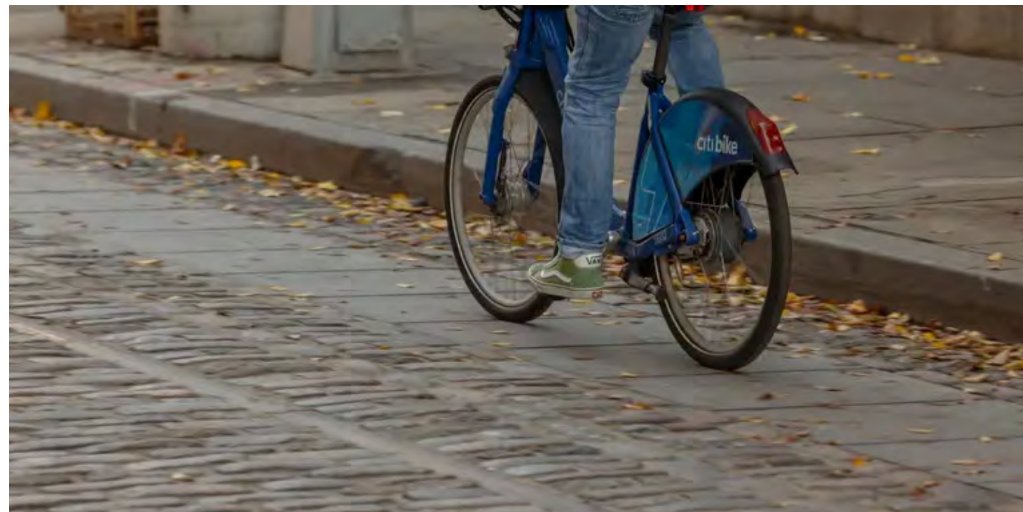
The road material should support a shared, safe, and sustainable streetscape and must calm vehicle and bicyclist speeds.
