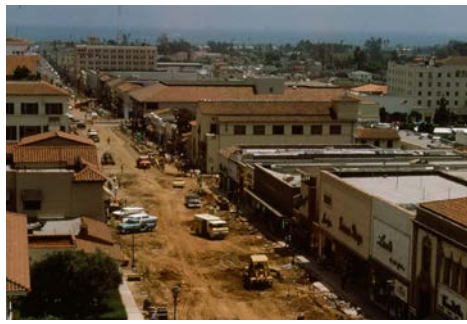
State Street, Under Construction
